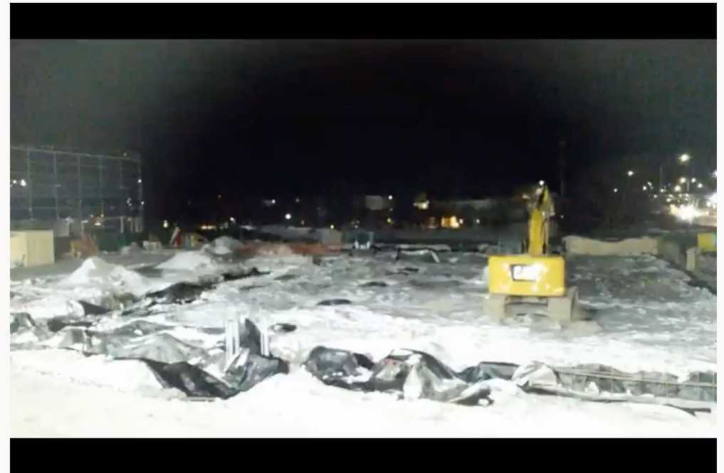
Pepper Construction case study
